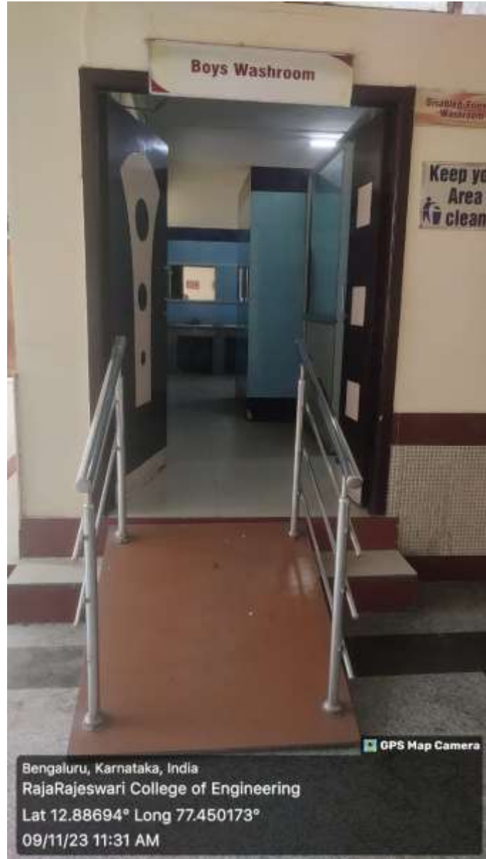
Photo.3: Disabled-friendly washrooms facility inside the college
