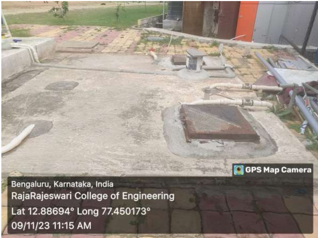
Photo.3: Water storage tanks in the campus
