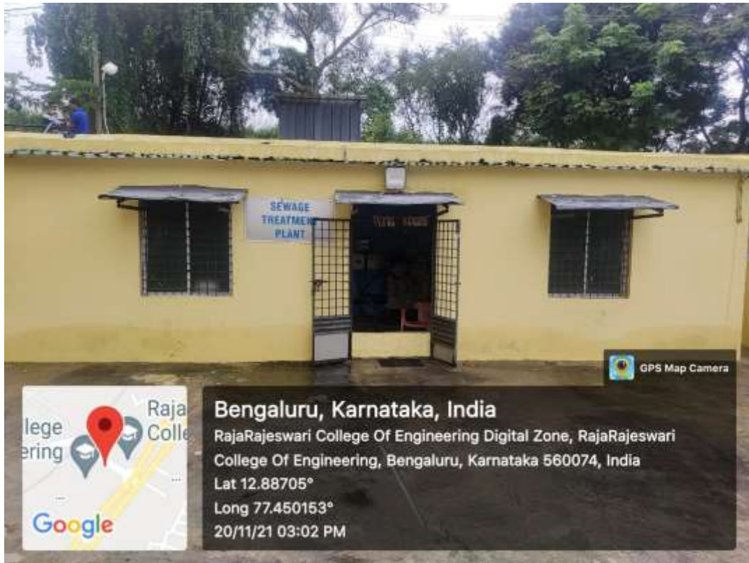
Photo.4: Centralized Sewage treatment plant at RajaRajeswari Dental College and Hospital (RRDCH)
